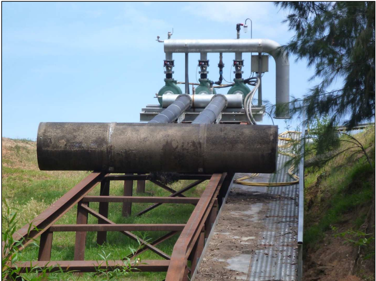
Figure 67. Example of a pump with screen.
