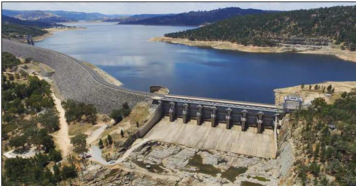
Figure 60. Wyangala Dam. Image courtesy Water NSW.
