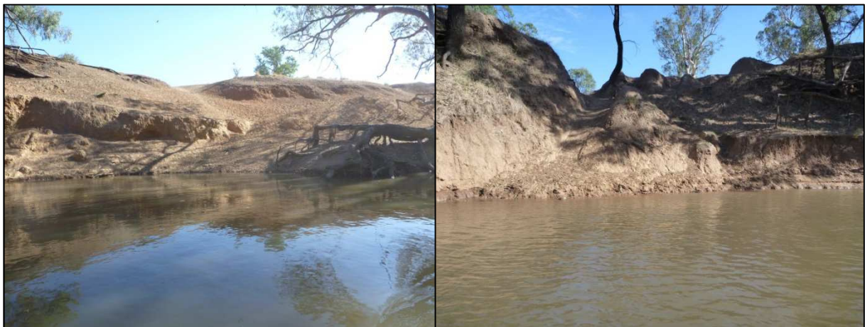
Figure 15. Damaged sites in the Lachlan River resulting from uncontrolled stock access.
